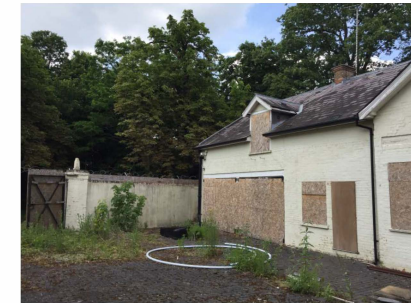
Precedent - Existing coach house (paint to be removed)
